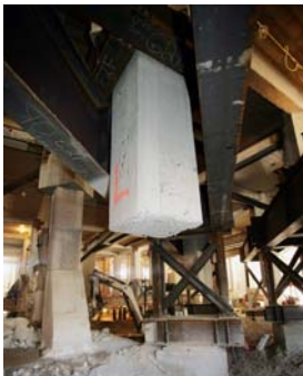
Old foundation column ready for installation of a base isolator
