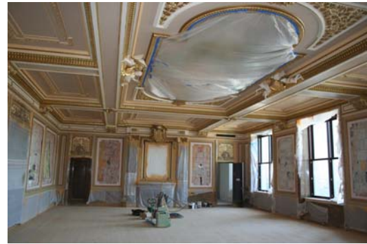
The State Reception Room under construction.
